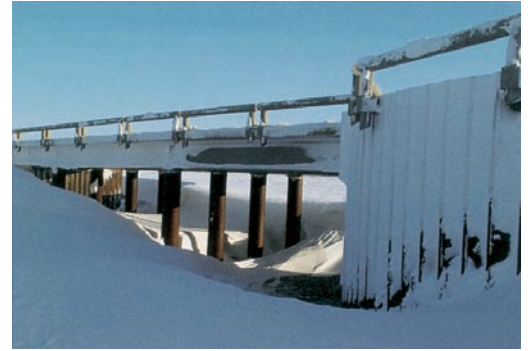
Open Cell Bridge - ConocoPhillips Alaska, Inc., North Slope, Alaska
